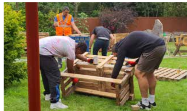
Bench construction at Reg's Garden, Farnborough station
