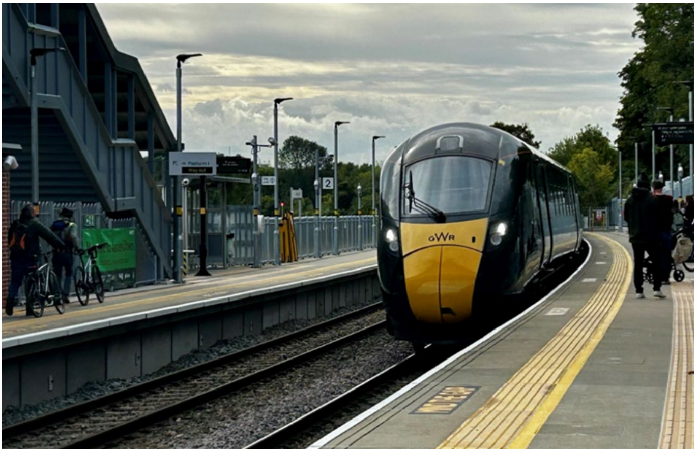
Ashley Down – one of the newly opened MetroWest stations
