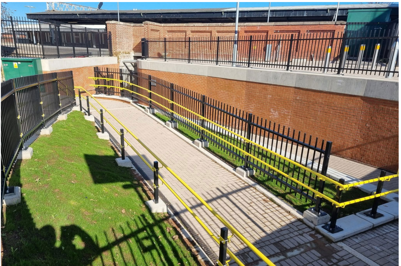
Step-free access to the underpass
